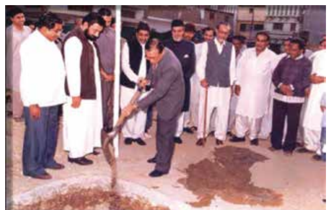
Foundation stone laying of Zainabia trust building
