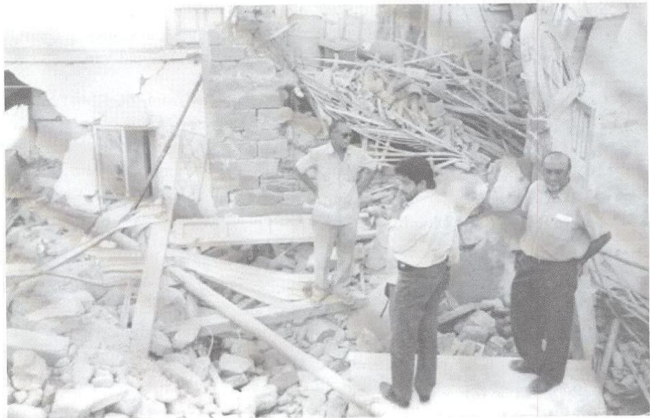
Extensive damage of Mehfil in Bhuj
