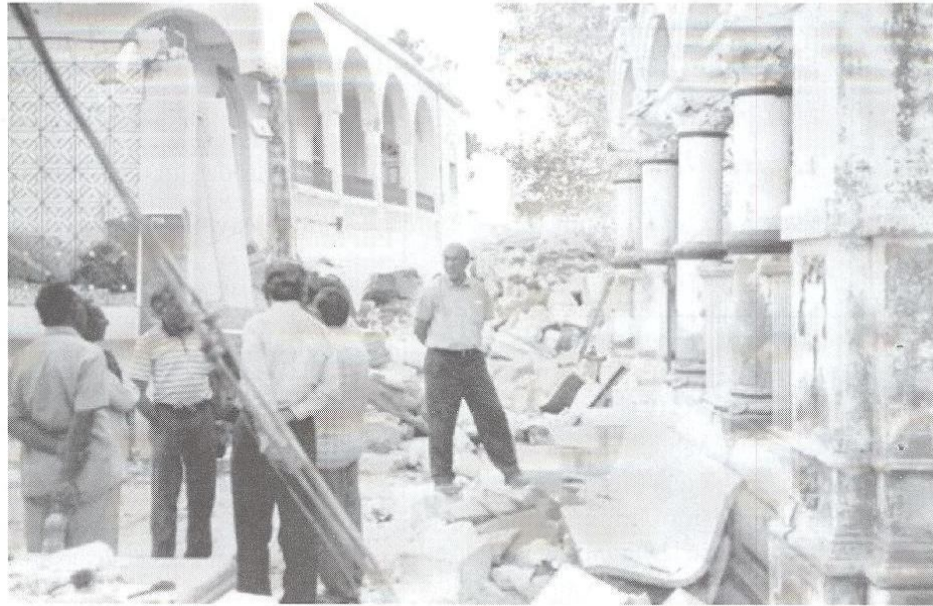
Surveying damage of Bhuj Imambara and Mosque
