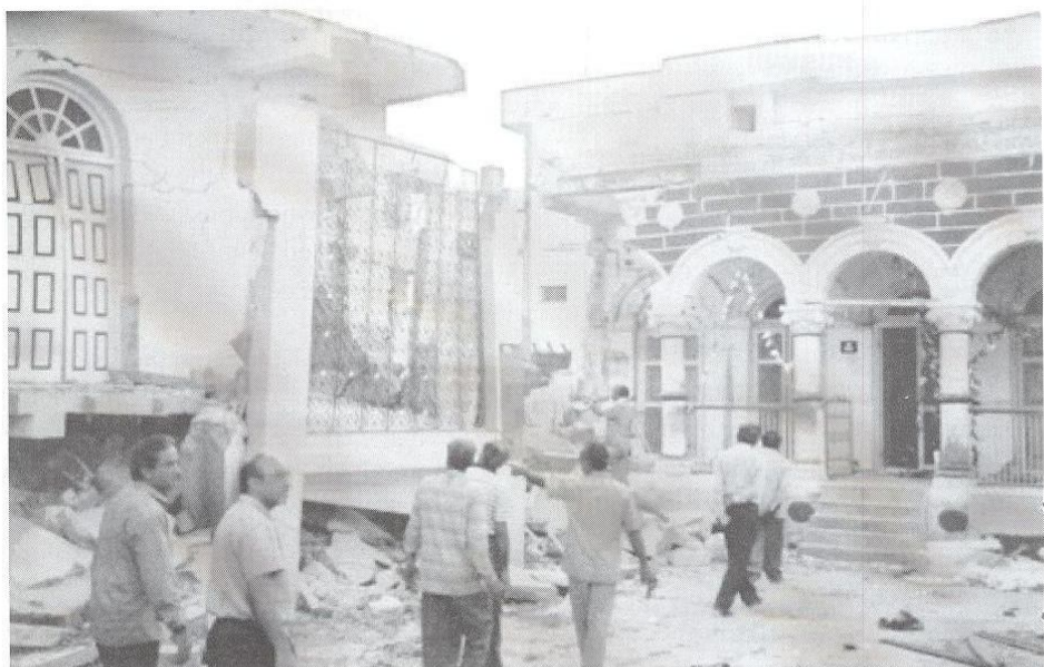
Damage of Bhuj Imambara and Mosque Complex
