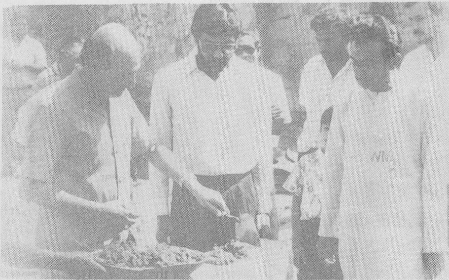
The Federation Chairman, Alhaj Habib Mulji laying the foundation stone to one of the proposed two buildings on Livingstone Road in Kariakoo area of Dar es Salaam. The President of Dar es Salaam Jamaat, Alhaj Aliraza Rajani and the Chairman of the CElebrations organising committee, Alhaj Roshan Fazal look on.
